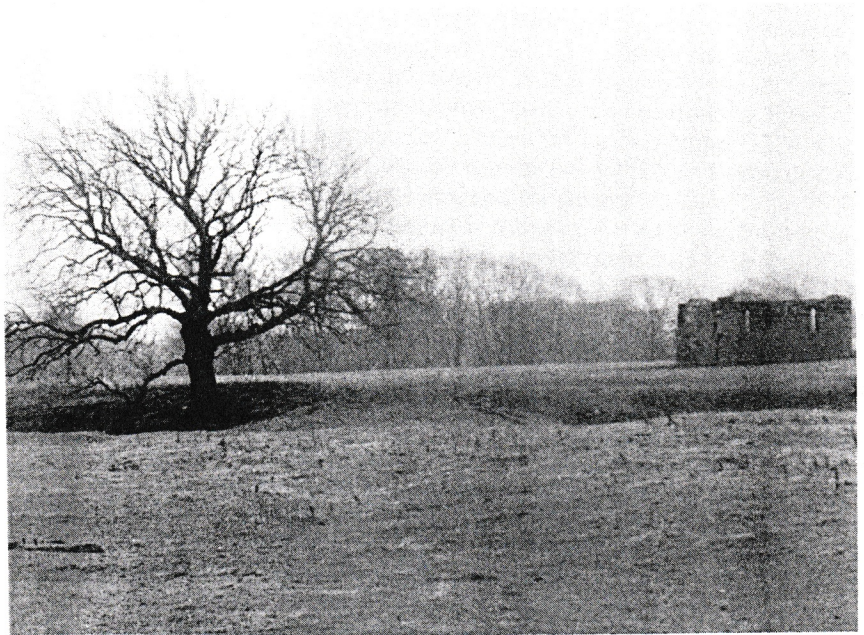
Two walls of its chapel are lonely evidence of the deserted medieval village of Cresswell
